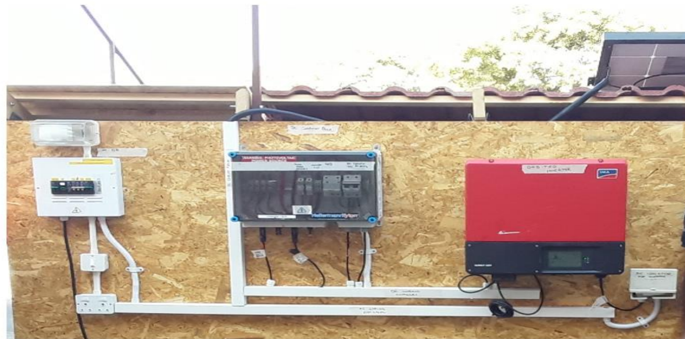
FIGURE 11: COMPLETED INSTALLATION TO BE ASSESSED
